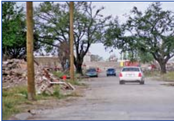
Repair work on Industrial Canal in distance, overlooking Ninth Ward.
