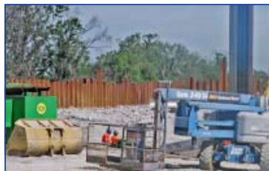
Working on the 17th Street canal
