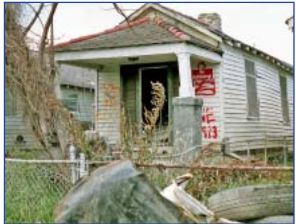
Note the NO BULLDOZING sign on the house of those expecting to return
